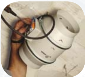
Carry out the wiring connections
