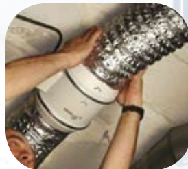
Connect the ducts
