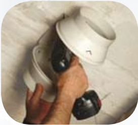
Fix the support bracket
