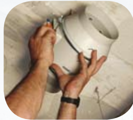
Place the impeller and motor assembly
